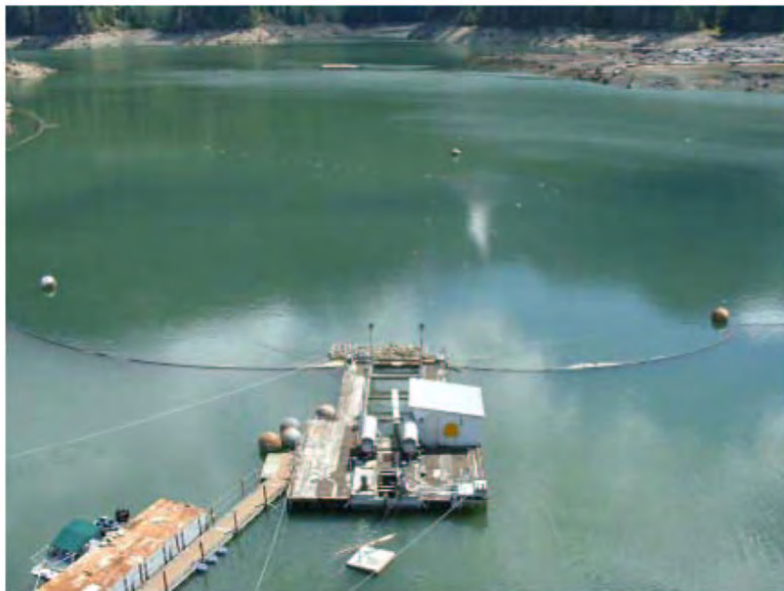
Figure 4-8 Gulper System in Use at the Baker River Fish Passage Project
