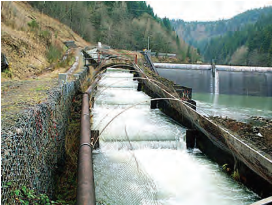
(b) The North Fork Dam fish ladder on the Clackamas River in Oregon, the longest (1.9-mile) operating fish ladder in the world.
