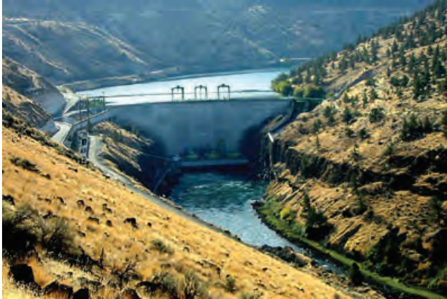
(a) A view of Pelton Dam on the Deschutes River in Oregon with fish ladder visible where it meets the dam on the left.
