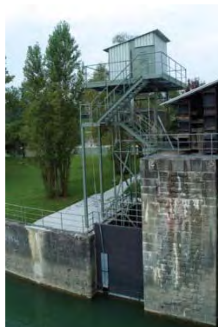
(c) A view of the fish elevator on the Connecticut River in Holyoke, Massachusetts.
